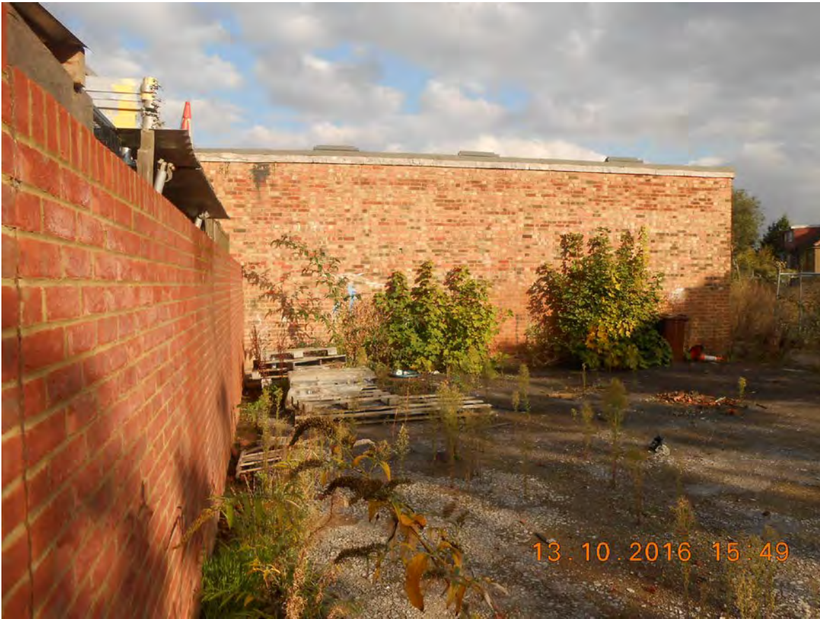
Existing single storey building used by Bailiffs
