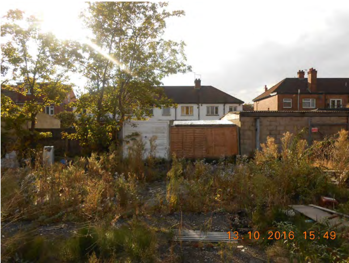
Rear elevations of adjoining properties along Harrow View
